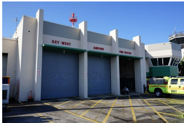
Exhibit 4.7-3: Aircraft Rescue and Firefighting Facility
